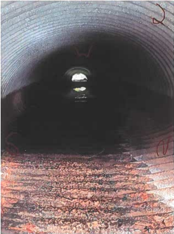
South Culvert Looking West
