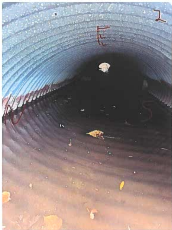
South Culvert looking East
