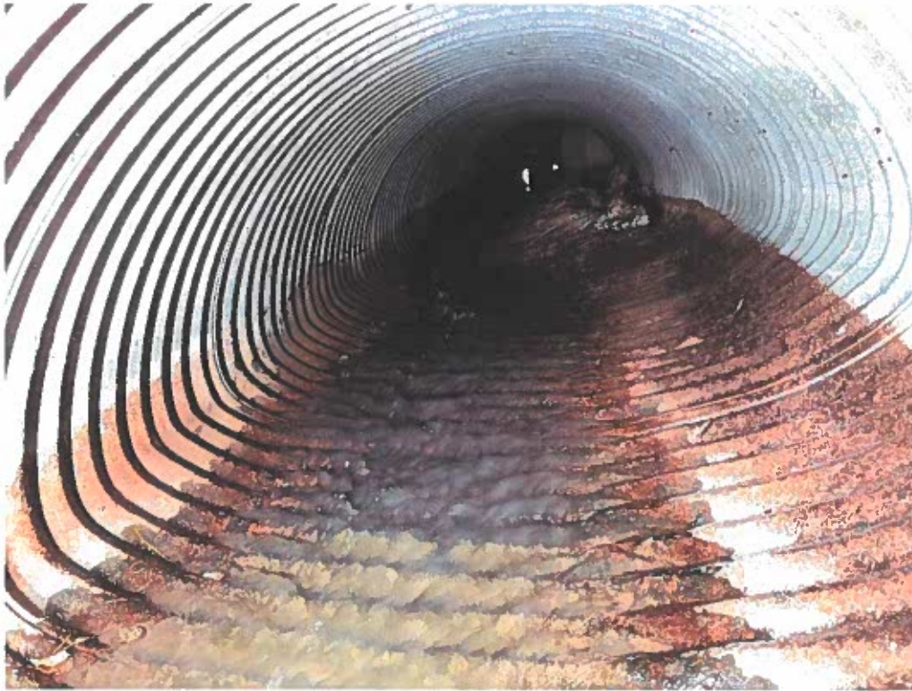
North Culvert Looking West – Notice bottom is buckled upward w/ obstructions.
