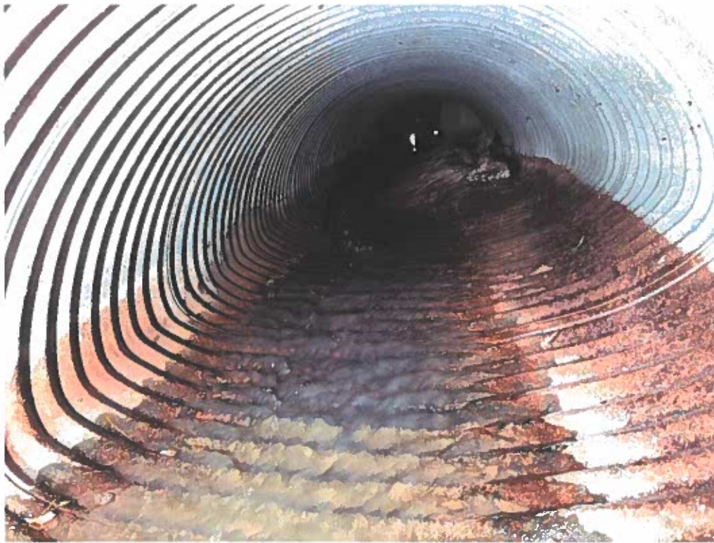
North Culvert Looking West – Notice bottom is buckled upward w/ obstructions.
