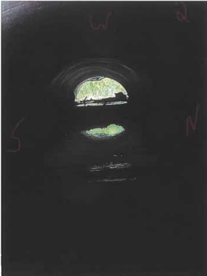
South Culvert looking West
