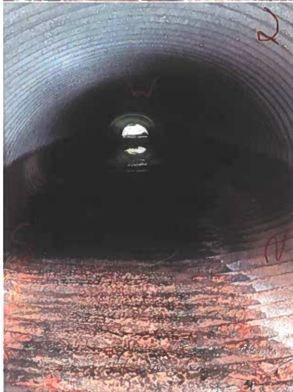
South Culvert Looking West
