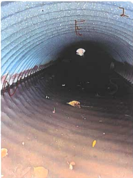
South Culvert looking East
