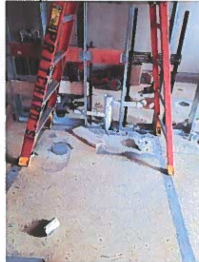
Women 204/Men 205 – Plumbing piping installation in progress.
