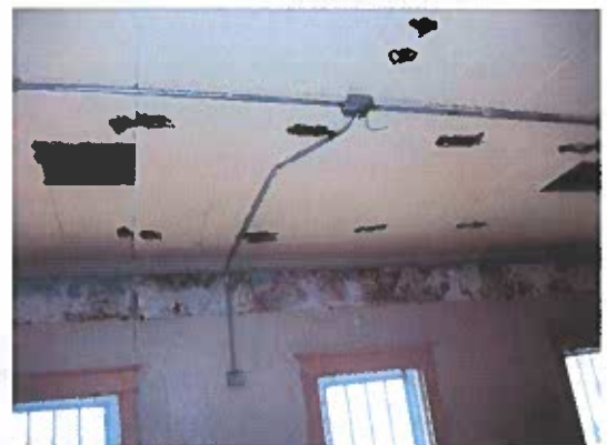
Multipurpose 201 – Conduit/box rough-ins
