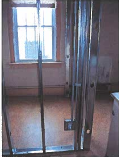
Jan 203 – Conduit/box rough-in
