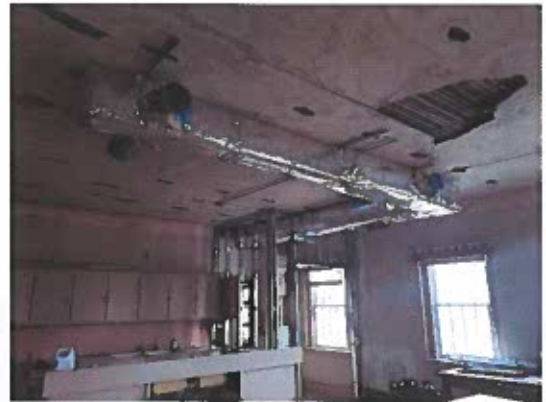
Staff Breakroom 202 ductwork rough in
