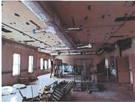
Multipurpose 201 ductwork rough in
