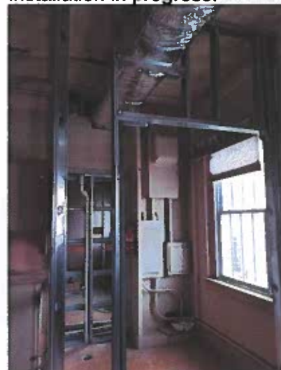
Janitor 203 ductwork and plumbing rough in
