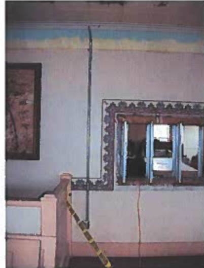
Multipurpose 201 – Conduit/box rough-ins
