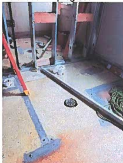
Women 204/Men 205 – Plumbing piping installation in progress
