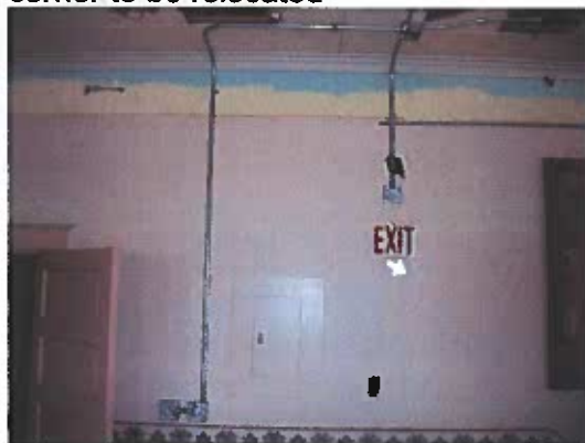
Multipurpose 201 – Conduit/box rough-ins
