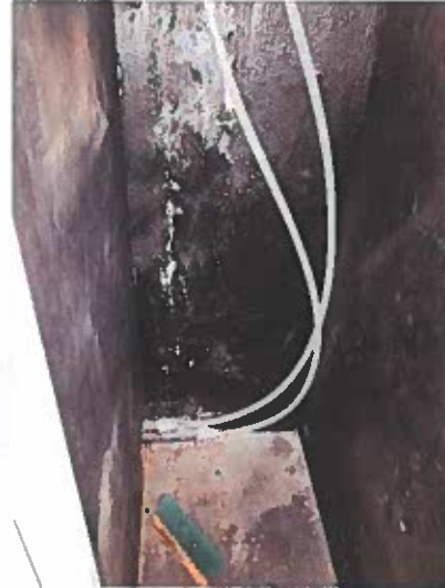
Unisex X110 - Domestic water piping to be replaced.
